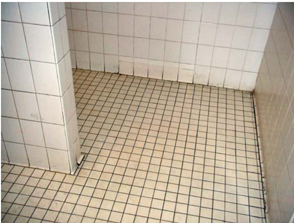
Discolored Tile Floor, Damaged Base
